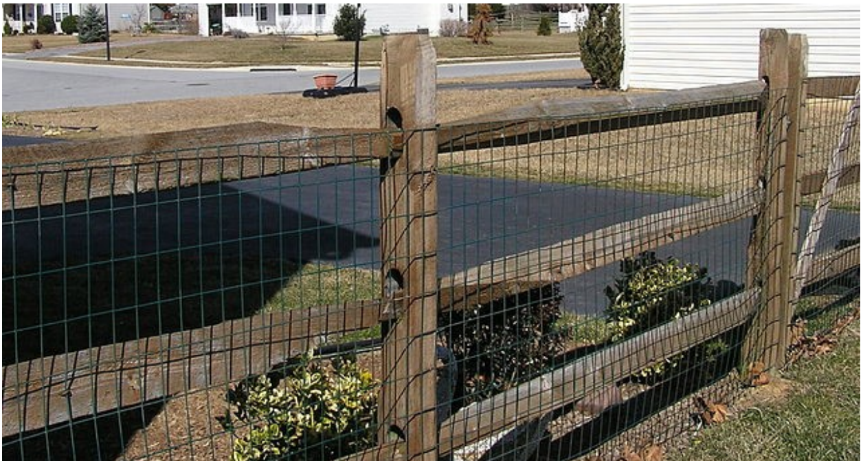
Example of Split Rail Fencing with metal mesh fencing attached
